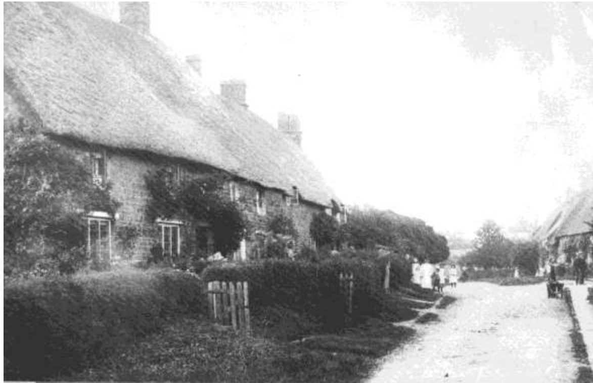
Looking up the High Street.
