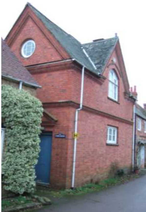
The Victorian Church Rooms
