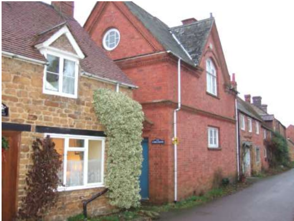
Left to right: 'Stone Cottage', Church Rooms and The Bakehouse
